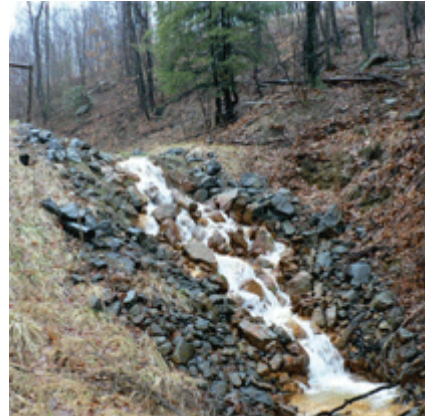
West Virginia must clean up toxic acid mine drainage from abandoned coal mines.
